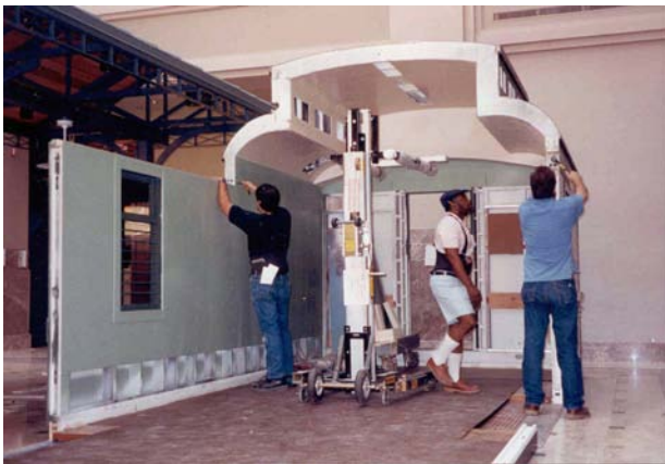
Smithsonian fabricators create the replica Railway Post Office sorting car on the NPM's exhibit floor. Although the car's interior furnishings are original, the museum's floor could not support the weight of the actual rolling stock. A lighter-weight copy had to be specially constructed.
